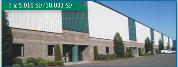
1155 Mid Valley Drive, Mid Valley Industrial Park, Olyphant, PA
