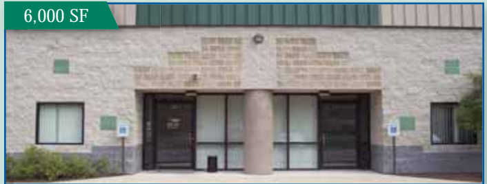
1125 Mid Valley Drive, Mid Valley Industrial Park, Olyphant, PA
