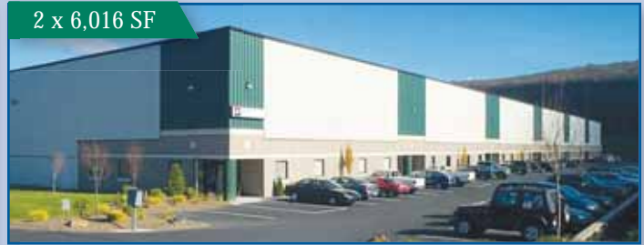
1175 Mid Valley Drive, Mid Valley Industrial Park, Olyphant, PA
