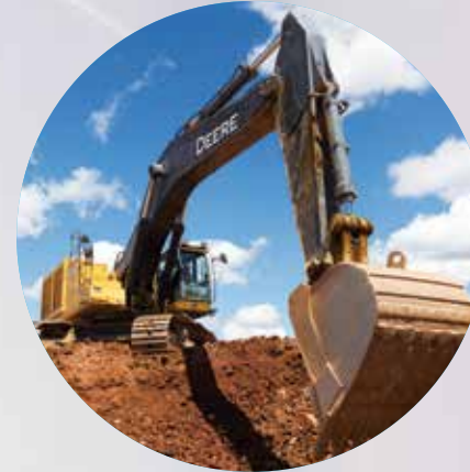
Mericle's 50 employee excavation division prepares ReadyToGo!™ Sites year round.
