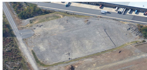
TECHNOLOGY DRIVE (PARCEL 26A) CENTERPOINT EAST | JENKINS TOWNSHIP, PA
